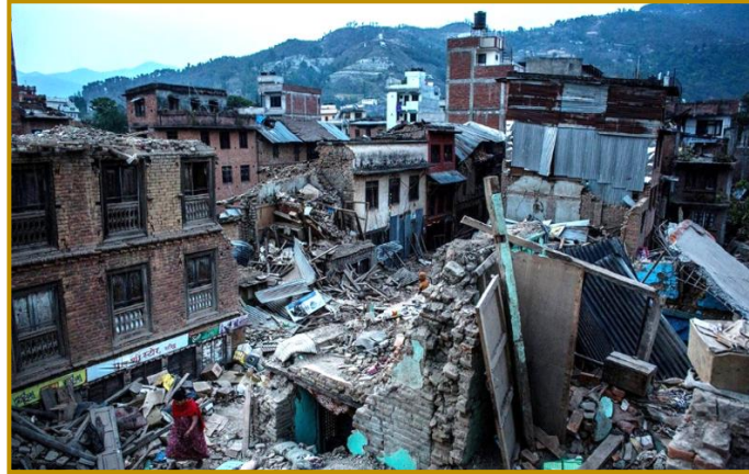
Figure of destruction caused by an earthquake
